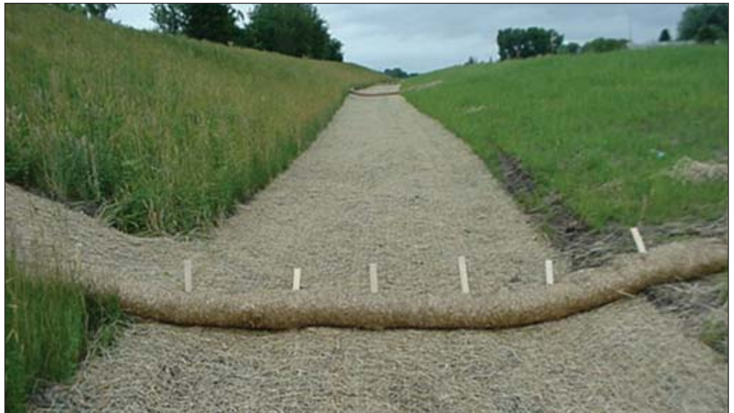
ABOVE: Erosion blankets are used to protect steep slopes and encourage vegetative growth. Photo courtesy of Allied Landscape
